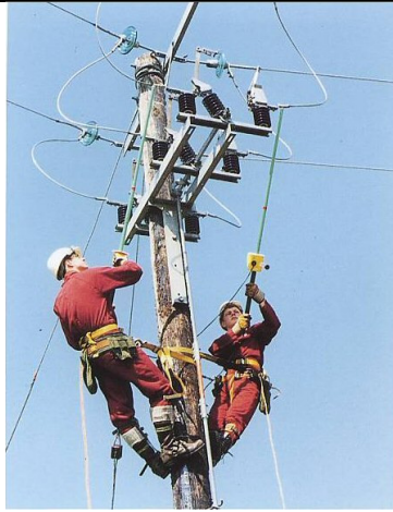
Overhead Line Testing
