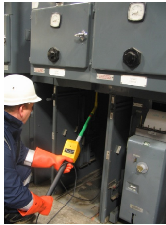
Switchgear Testing
